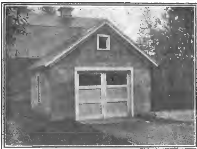
Dr. Best's garage at Englewood, N. J. This is built of concrete and cost $445
